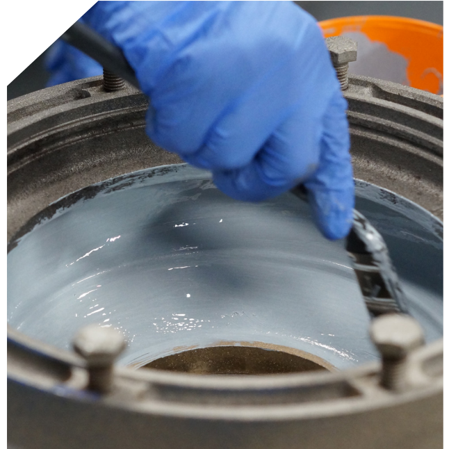
Belzona coatings are applied by experienced engineers in a controlled environment at our Dudley workshop.
