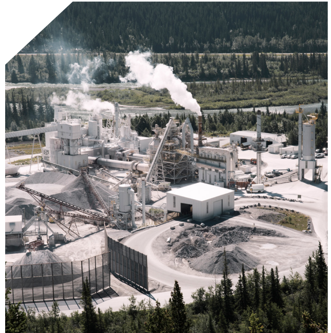
Cement plants and other environments handling raw materials are some of the toughest for bearings.
